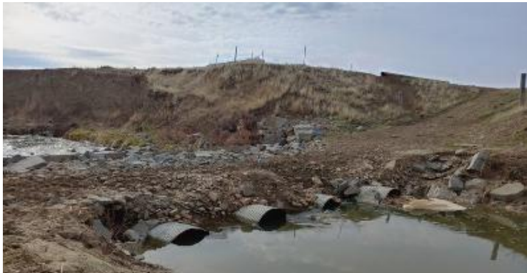
Pre-project conditions showing the old crossing with undersized culverts and unrestricted cattle access.
