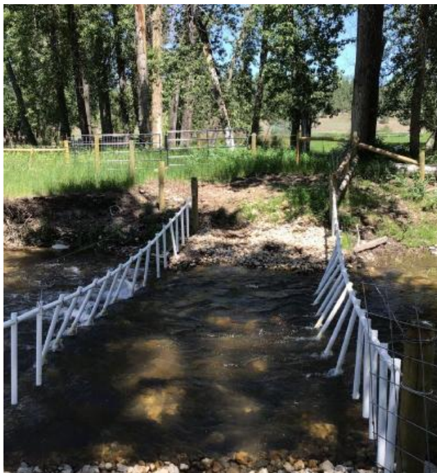
Example of a water gap to limit livestock access and reduce impacts to water quality (photo by Bitter Root Water Forum).
