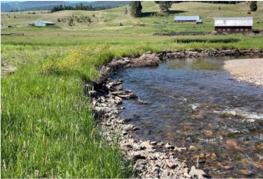
Post-project photo showing successful restoration work to reduce streambank erosion on Nevada Creek (photo by BBCTU).
