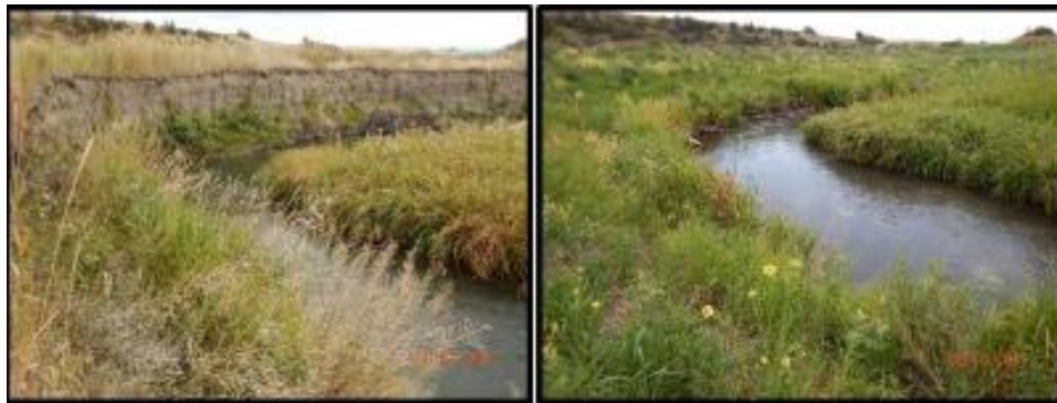
Pre-restoration photo from 2018 (left), compared to a post-restoration photo from 2019 (right), showing restored and revegetated streambanks from the 2019 phase 2 project on a nearby section of Dry Creek (photo by Trout Unlimited)
